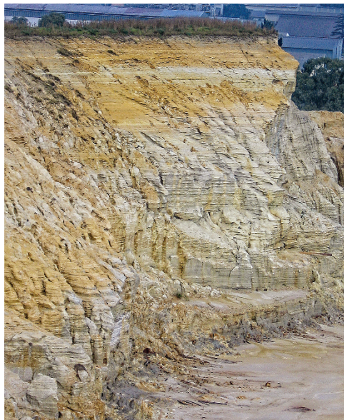
Figure 4.2 Exposed mature oxidation zone (MOZ) with underlying Transitional Zone (TZ) (TSF5) with a vegetation cover on top.
